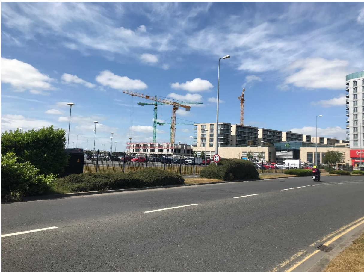
Plate 3.2: View North West Across the Site from St. Margaret's Road
