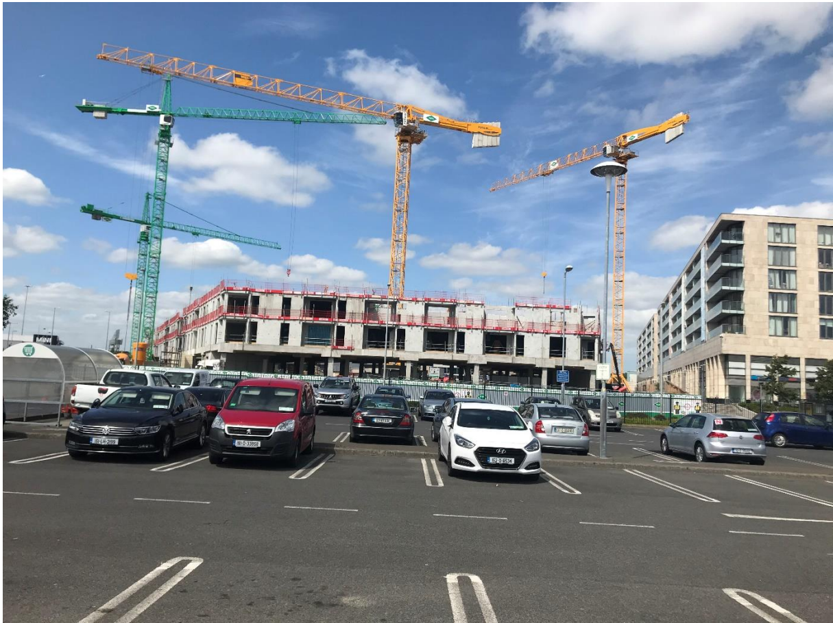
Plate 3.9: View North from the Centre of the Site
