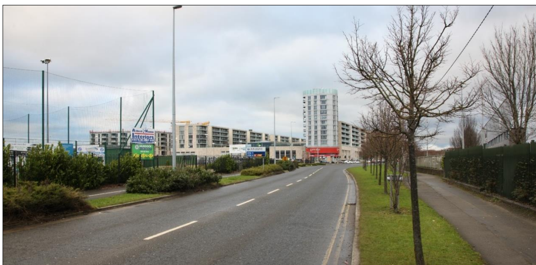
Figure 14.7: A view from St Margaret's Road approaching the town centre with the McKelvey Celtic football club and the site in the foreground to the left. Note the urban character and the architectural and material quality of the Charlestown Centre buildings
