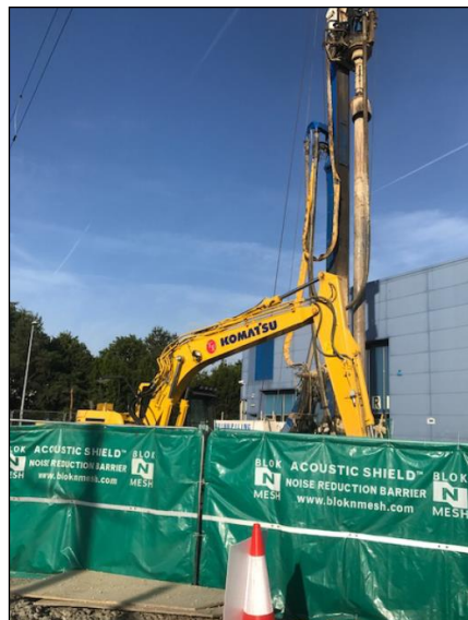
Acoustic blankets screening piling and excavations
