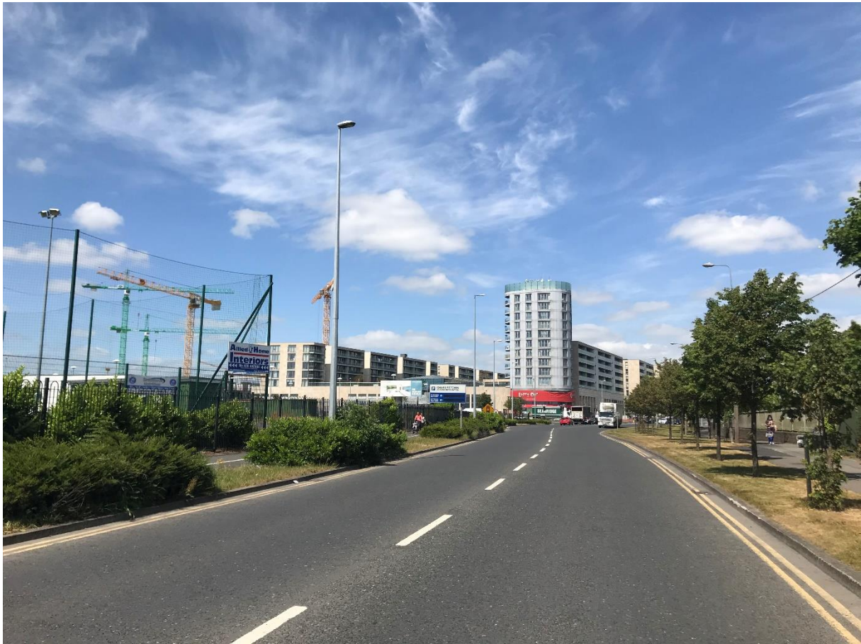
Plate 3.1: View North Towards the Site from the South on St. Margaret's Road
