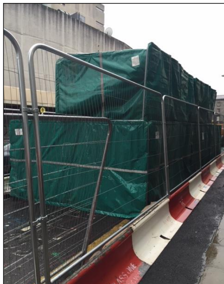
Double height acoustic blanket enclosure
