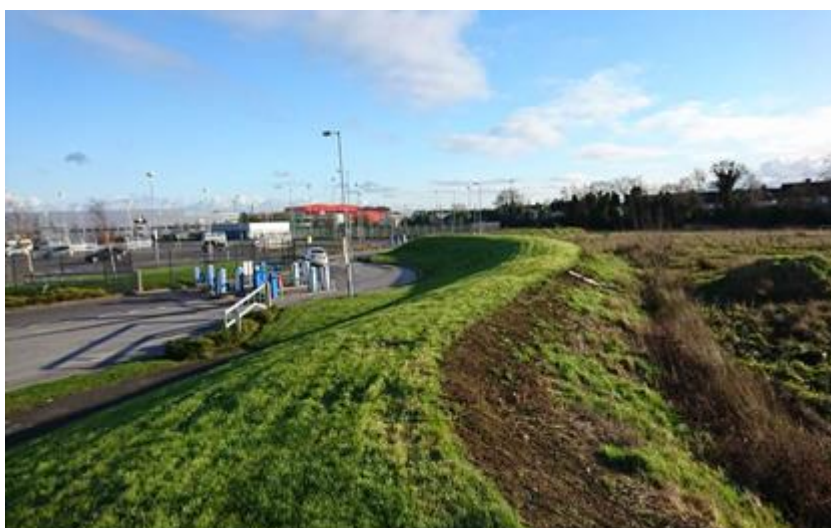
Plate 13.3 Road to car park and berm in western portion, facing southeast
